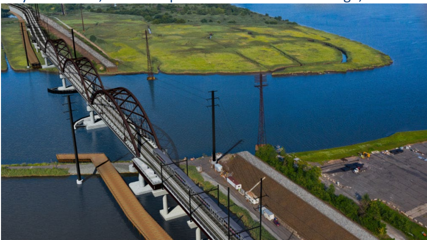
Aerial rendering of the new Portal North Bridge, courtesy of the NJ Governor's Office
