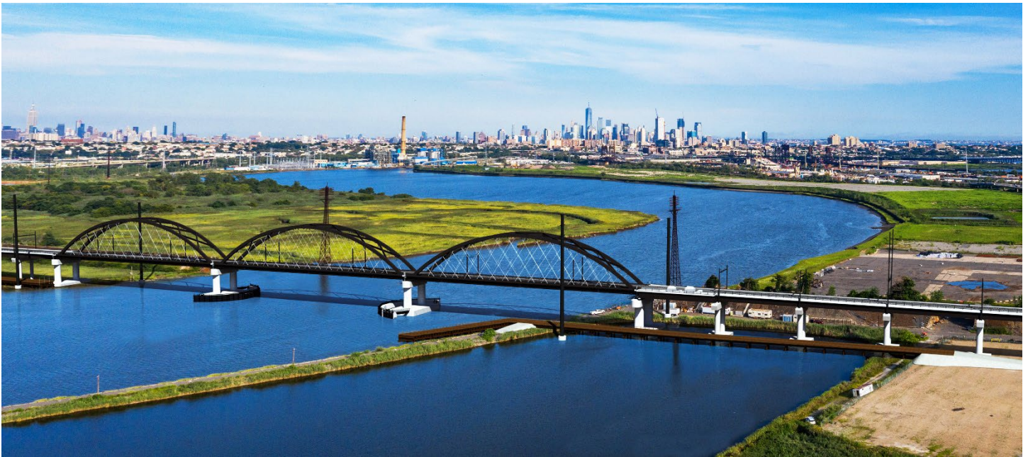
Portal North Bridge replacement in Hudson County, New Jersey
